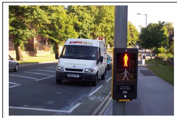
PDU in foreground with approaching traffic in the background
