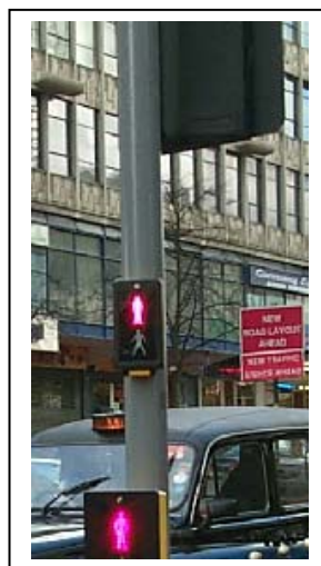
Smaller high level repeater under trial
