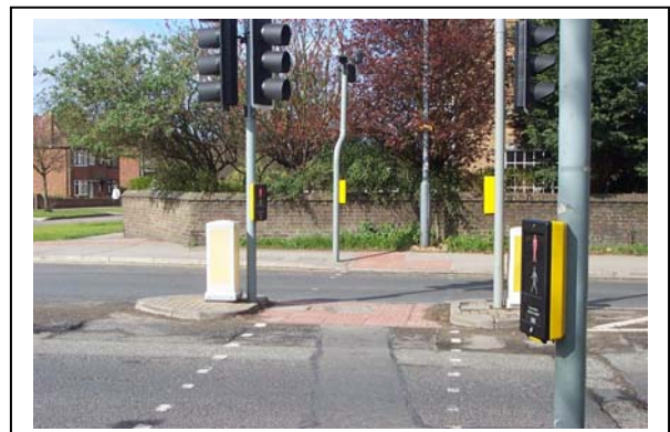
PDU's on refuge incorrectly aligned
