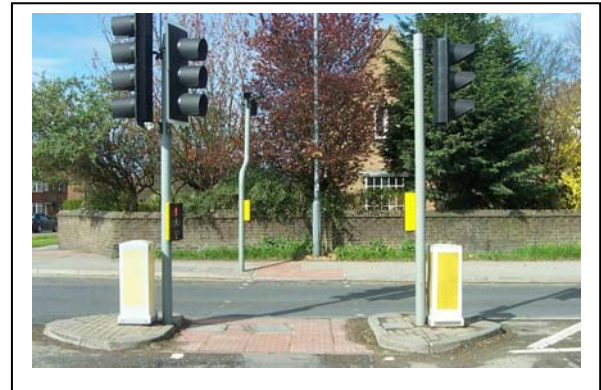
PDUs on central refuge area incorrectly aligned
