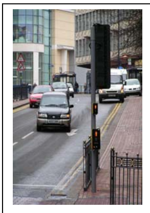
High level repeaters
