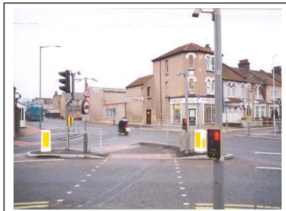
Puffin crossing at junction traffic signals
