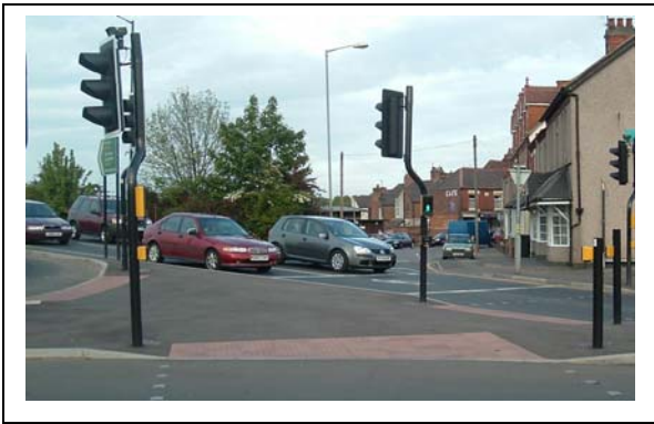
See-through at junction traffic signals
